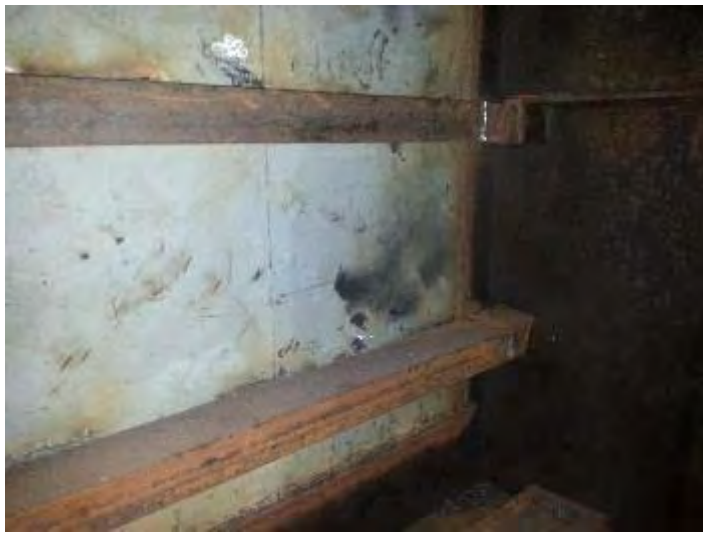
SHELF DRILLING JACK-UP RIG RANDOLPH YOST SIDE SHELL REPAIRS
